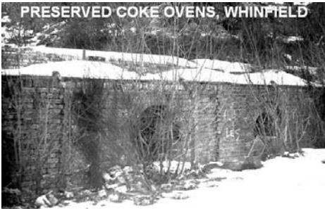
PRESERVED COKE OVENS, WHINFIELD
